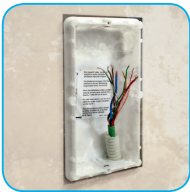
Removal of the existing entrance panel
