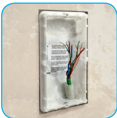
Removal of the existing entrance panel
