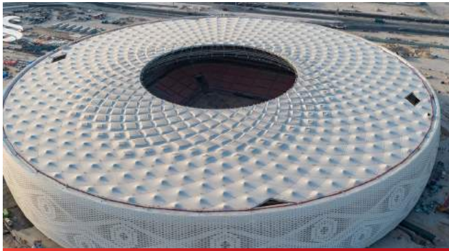
Al Thumama Stadium Qatar
